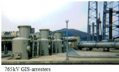
Fig.8 Outside View of 765kV GIS-arresters (10)
