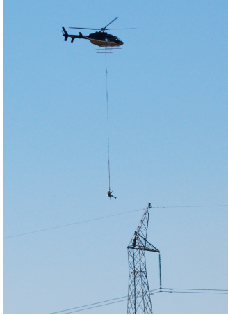
Figure 1: Live worker being lowered onto the conductor
