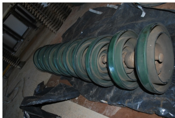
Figure 1: Removed insulator strings - Tower 122.
