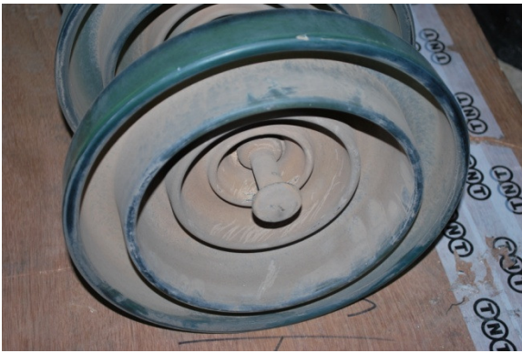
Figure 2: Removed insulator strings - Tower 119.
