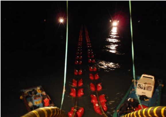
Figure 14: Simultaneous Cable Laying
