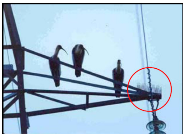
Figure 7: Perching guard needle type [5]
