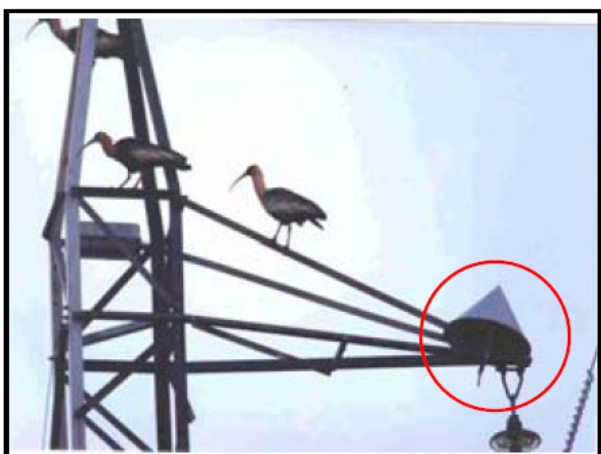
Figure 6: Perching guard cone type [5]
