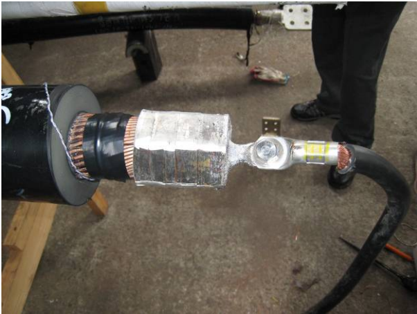
Fig 7. Soldering method
