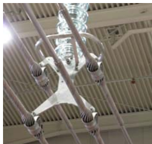
Figure 2b: Close-up View of the single “I” suspension string assembly
