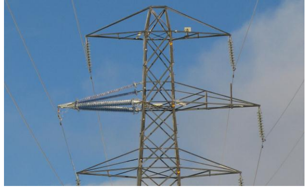
Figure 8: Completed retrofit installation of composite cross-arm
