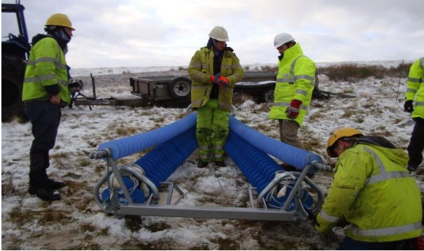
Figure 5: Assembling the composite cross-arm
