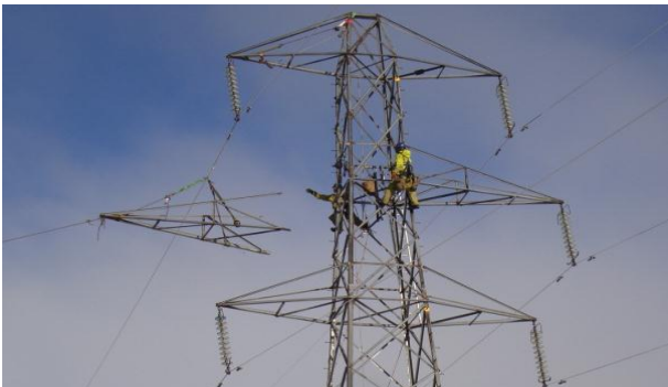
Figure 6: Removing the metallic cross-arm
