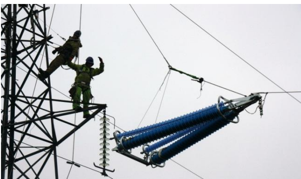
Figure 7: Raising the composite cross-arm
