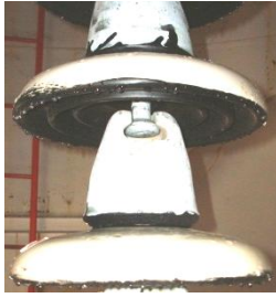
Figure 1: coating applied to the pin area
