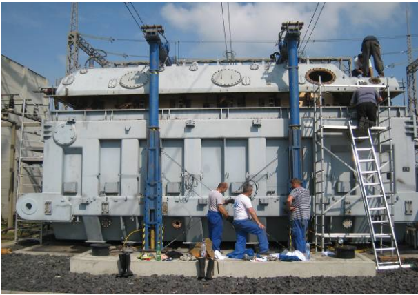
Figure 1: Un-tanking with CRAB lifting system
