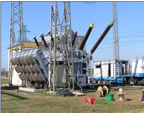
Figure 3: On-site induced HV test on transformer
