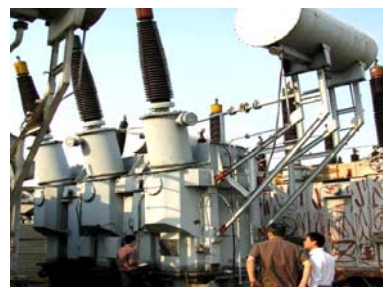
(a) The transformer under test
