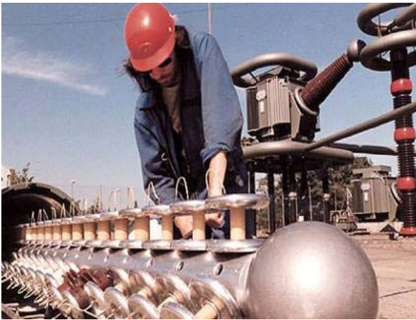
Figure 5: Example of a long-term high-voltage test setup
