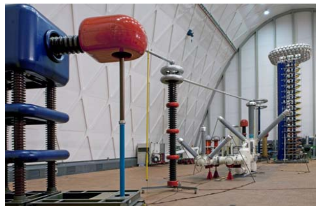
Figure 4: Example of a high-voltage type test of a 145 kV GIS in the high-voltage laboratory
