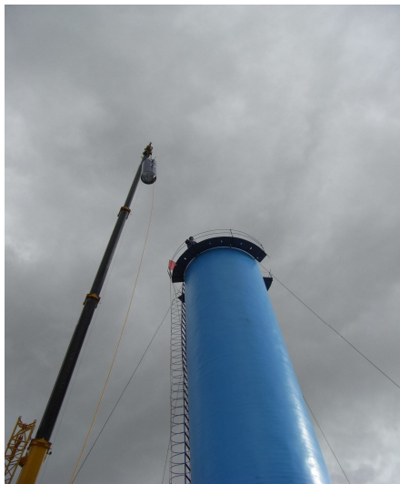
Fig 3 Hoisting of impulse generator
