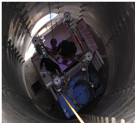
Fig 4 Installation of impulse generator
