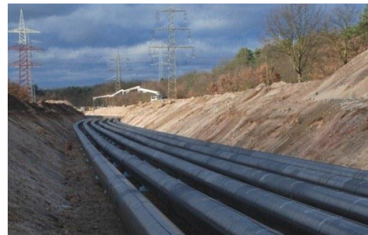
Figure 1: Trench with GIL phases
