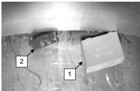
**Figure 9:** The capacitor (1) and resistor (2) connected parallel to the gap between resonator and inner conductor of GIS
