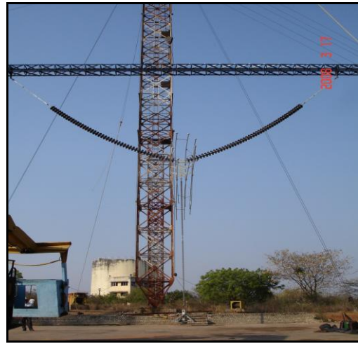
Figure 4: A view showing 1200 kV Single 'V' string suspended from a cross-arm.
