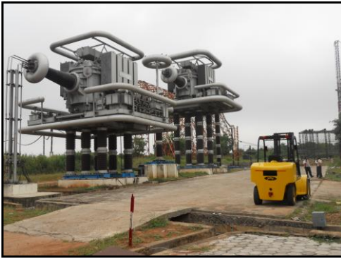
Figure 3 : A view of the 1600 kV Test transformer along with the divider.
