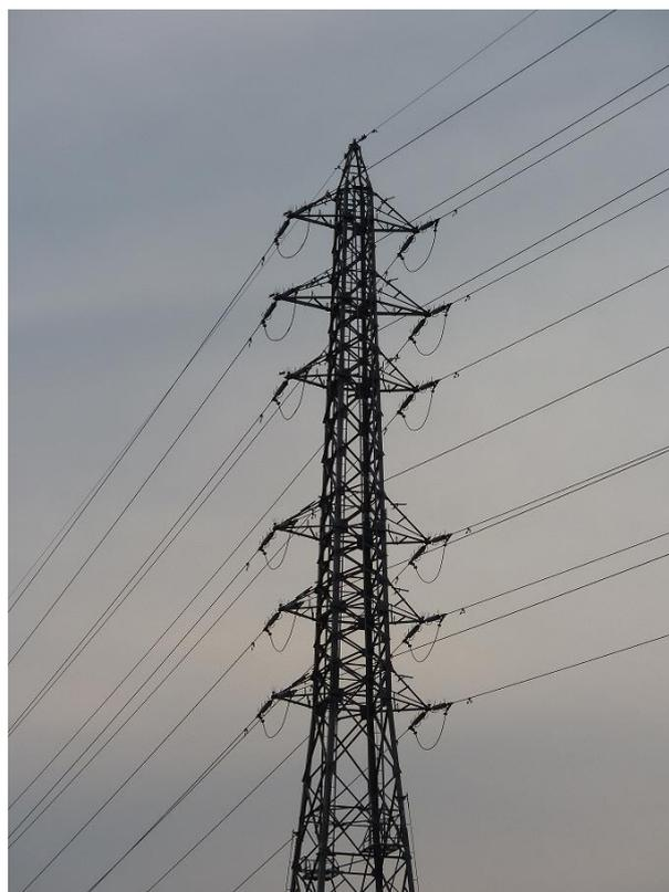
**Figure 1:** Vertical-type two double-circuit power lines
