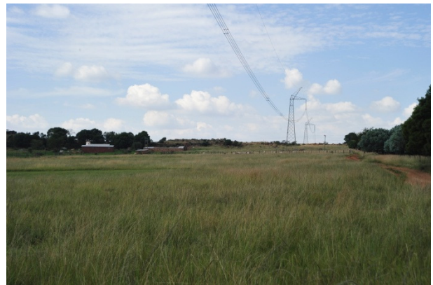
Figure 9: Measurement site under Cahora-Bassa 533 kV line (Positive monopole)
